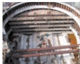
LEFT CTRL Contract 250; the chamber for installation of the two tunnel boring machines; both permanent and temporary works designed by Kier Engineering Services.
