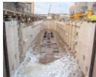
LEFT Major dock upgrade at Devonport Dockyard. Kier Construction.
