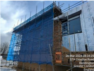
Brickwork and scaffold ongoing.
