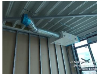
Heating and cooling units in classrooms being installed.
