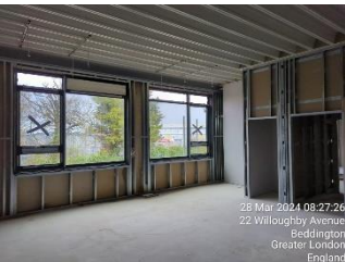
Windows installed and internal walls being constructed.
