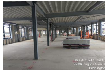
Plasterboard being loaded out for internals to start.
