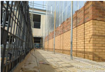
Brickwork to sports hall ongoing.
