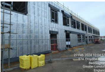
SFS insulation around the building ongoing.
