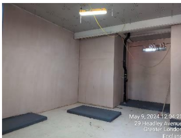
Plant room construction.
