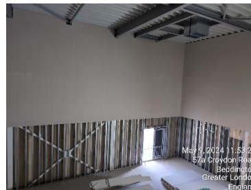
Boarding of sports hall, containment to follow.
