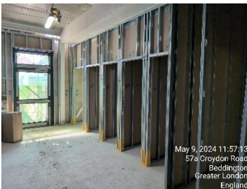
Construction of toilets throughout building.
