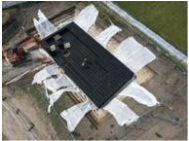
Installation of Site Soak Away Drainage
