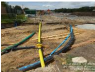
Water, gas and fibre optic ducting and pipework installed.
