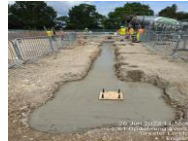
Commencement of pad foundations
