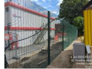
Permanent fencing was erected to the east elevation
