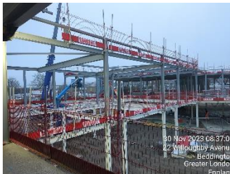
Phase 3 steel work installed.
