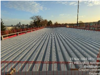
Phase 1 roofing deck complete.
