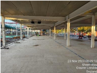
Phase 1 slab pours completed.
