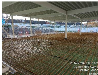
Phase 2 waterproofing and mesh install, ready for concrete pour.
